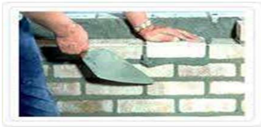
Figure 1: Application of mortar
